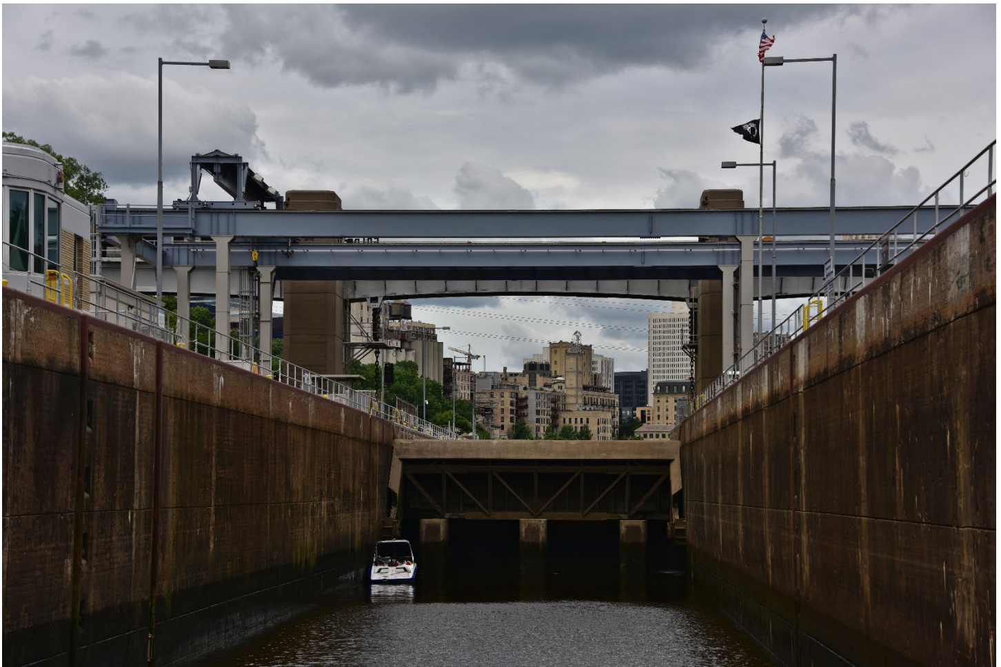
Lower St. Anthony Falls Dam, Mississippi River; Photo Credit: August Schwerdfeger [flickr]
