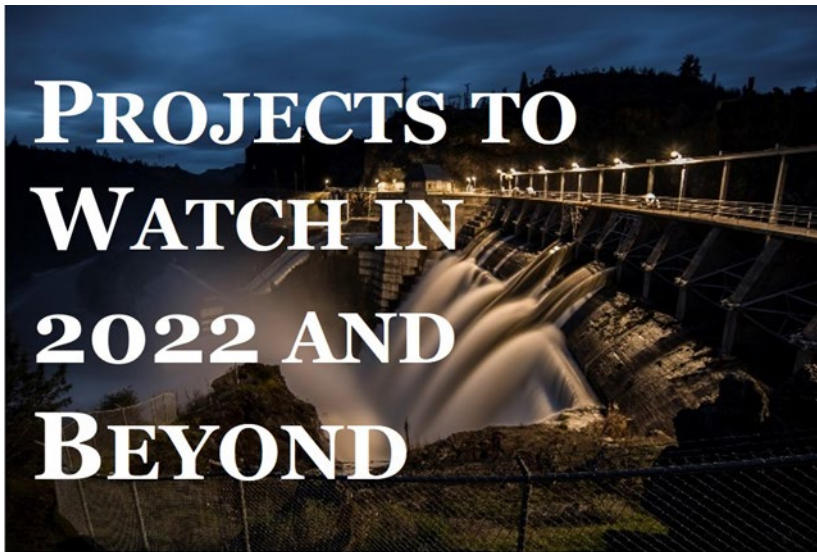
Copco 1 Dam, Klamath River; Photo Credit: Daniel Nysten
